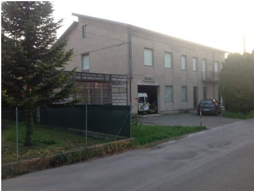
view from north-east
