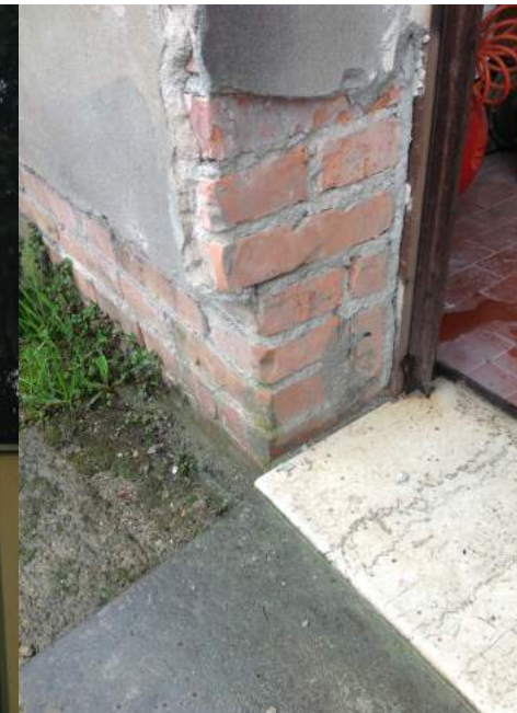
detail of masonry
