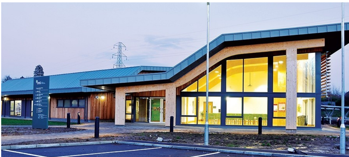
Figure 1: The CREST Pavilion with design featured solar control in brise-soleil and large overhangs.
