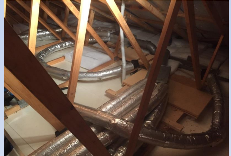
Insulated ductwork outside thermal envelope
