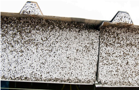
EPS roof insulation (200mm, U = 0.20 \text{ W/m}^2\text{K} )
